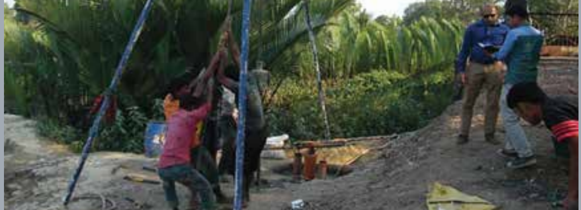
Figure 5: Soil investigation of Balikhali- Gundhum construction project, Cox`s Bazar
