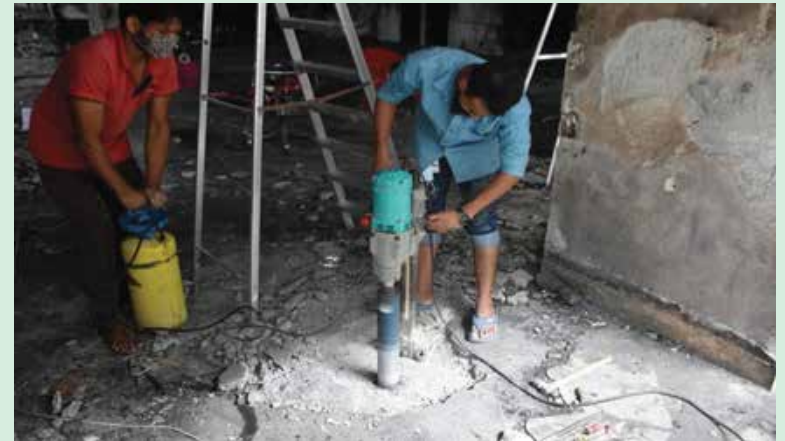
Figure 1: Core collection from FR Tower, Banani, Dhaka
