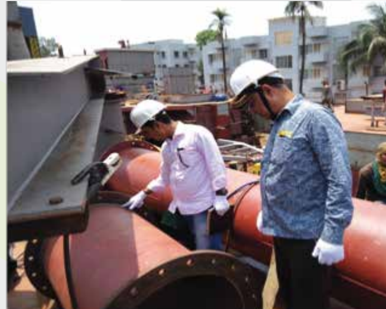
Figure 1: Inspection of discharge pipes and floaters of dredgers
