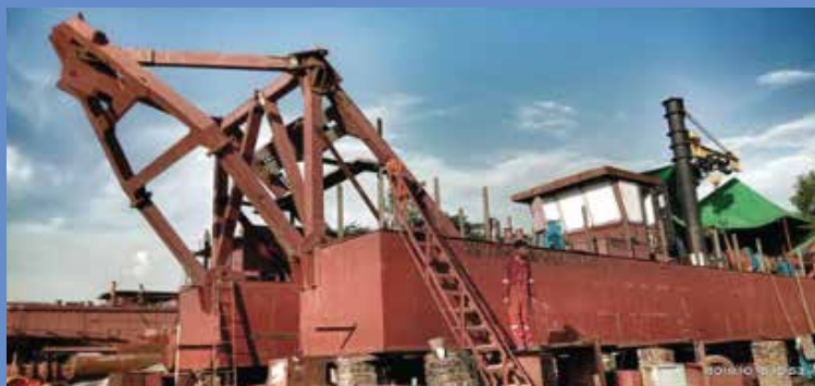
Figure 9: Construction of dredger for CPA
