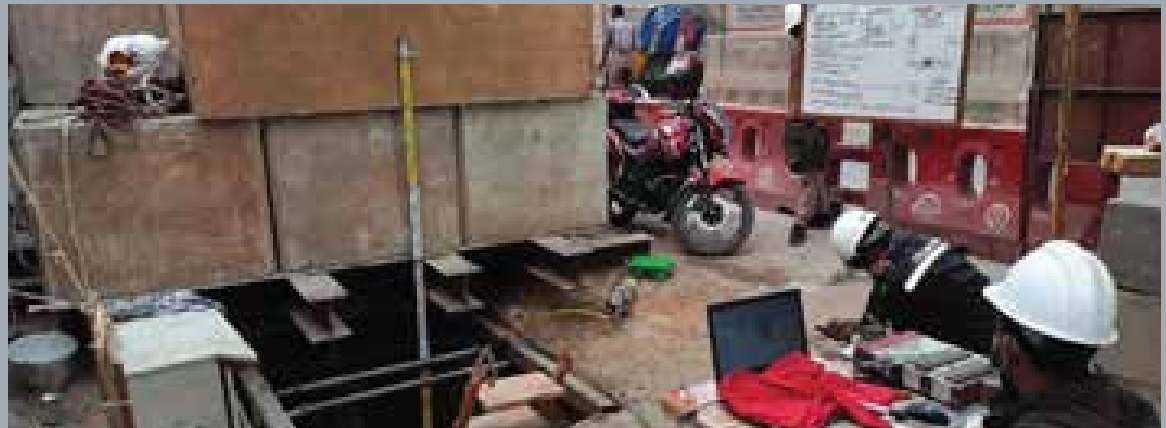
Figure 6: Mass rapid transit (MRT), plate load test, station 9
