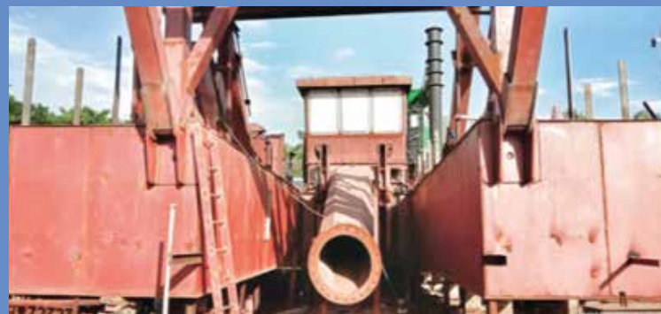
Figure 10: Dredger under construction
