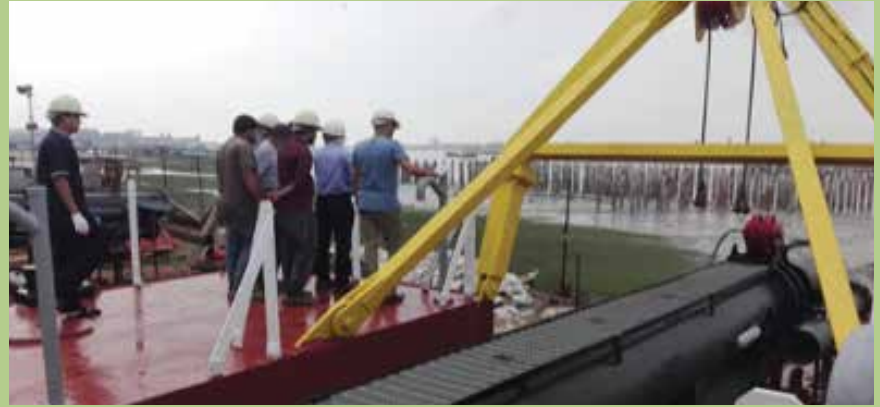
Figure 3 - Inspection of the cutter ladder and gantry crane of dredger 450 mm
