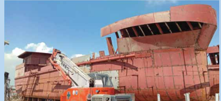
Figure 7: Self-propelled Water Barge construction in Karnafuly Dockyard, Chattogram
