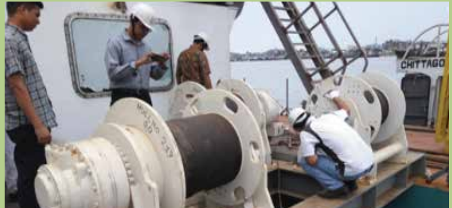
Figure 4: Inspection of ladder winch installation of dredger 650 mm
